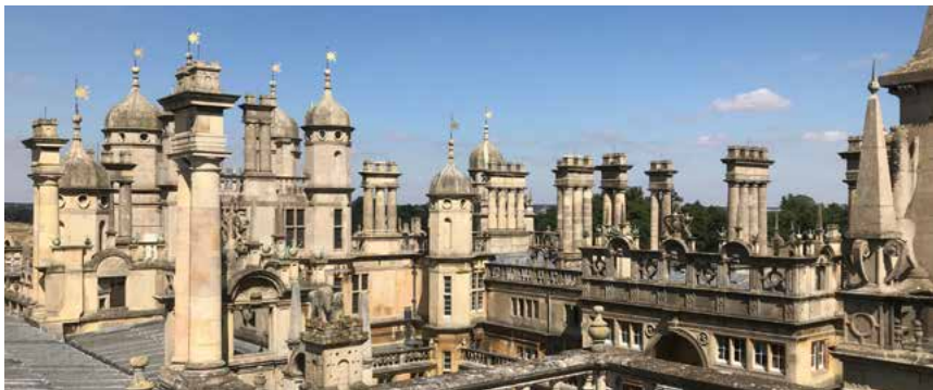
Figure 4.26.1 Burghley house, "Burghley House Roofline" (Digital photograph, 2019). © Burghley House Preservation Trust Limited.
