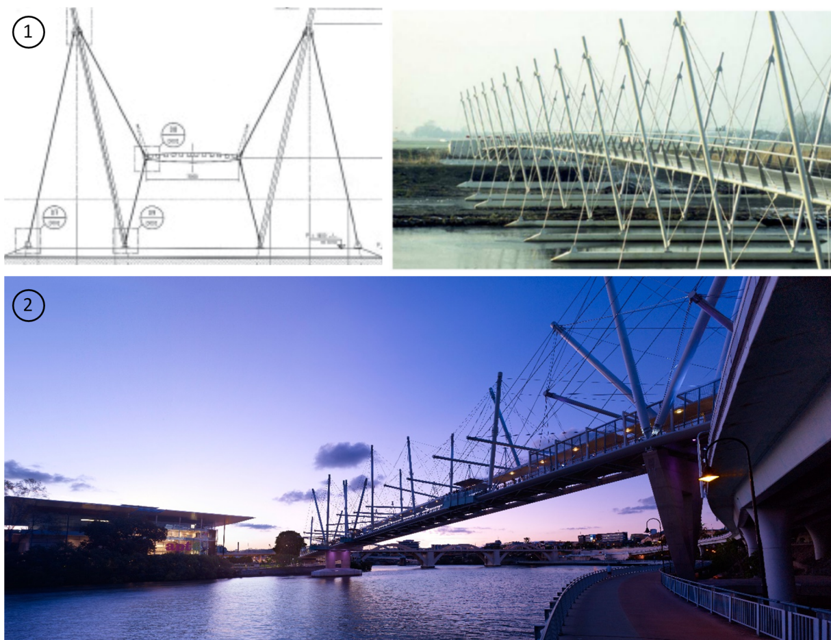
Fig. 2. Existing footbridges: 1 - Bridge of Masts (2000, Purmerend, Netherlands) by den Hollander (Eekhout, 2016, reprinted with permission), 2 - Kurilpa Bridge (2009, Brisbane, Australia) by Cox Rayner Architects and Arup.
