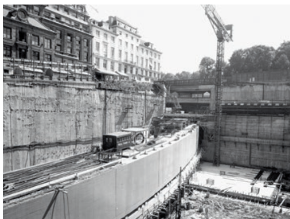
Construction of the metro between Parc and Gare Centrale stations during the work on the BNP Paribas Fortis headquarters at Montagne du Parc, 1969.
