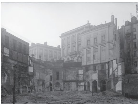
Retaining wall in Rue Isabelle during construction of the Centre for Fine Arts (BOZAR), 1911.
