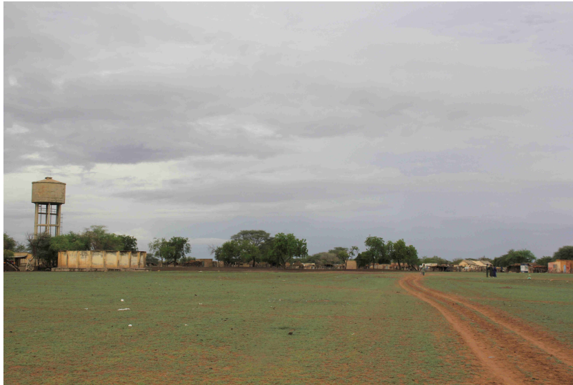
Figure A2.8 – Deep well of Widou Thiengoly. On the left, the hydraulic pump and the water tank. On the right, Widou village. Photo: M. Dendoncker, August 2015.
