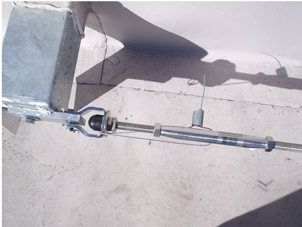
Figure 4: Anchorage mechanism (Point C in Figure 1).
