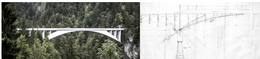
Fig. 1 Salginatobel Bridge (1929) from Robert Maillart. Left: picture taken by D. Zastavni (2022). Right: graphic static drawing: with form diagram on the right.
