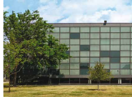
Keating Hall at the Illinois Institute of Technology by Myron Goldsmith, Chicago, Illinois, USA. Ph. Jonathan Choe
