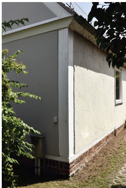
Fig. 4: Left: Detail of "T 4" house built with Patentwand wall system conceived by Heinrich Tessenow, Gartenstadt Hellerau, Dresden. Right: Heinrich Tessenow, drawings of the Patentwand wall system and original pictures of the Patenthaus construction
