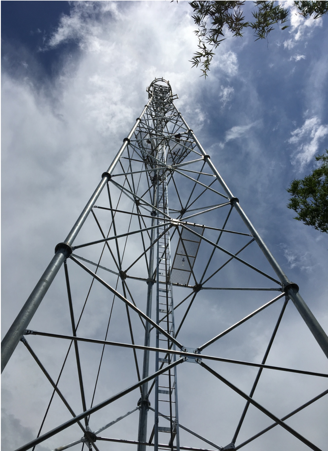
Picture 3.8. This cellular tower of one of the major telecom companies in the Philippines was being constructed just behind the house where I stayed during my fieldwork on Talim Island in 2017. Photo: Angelito Nunag (25 May 2017).
