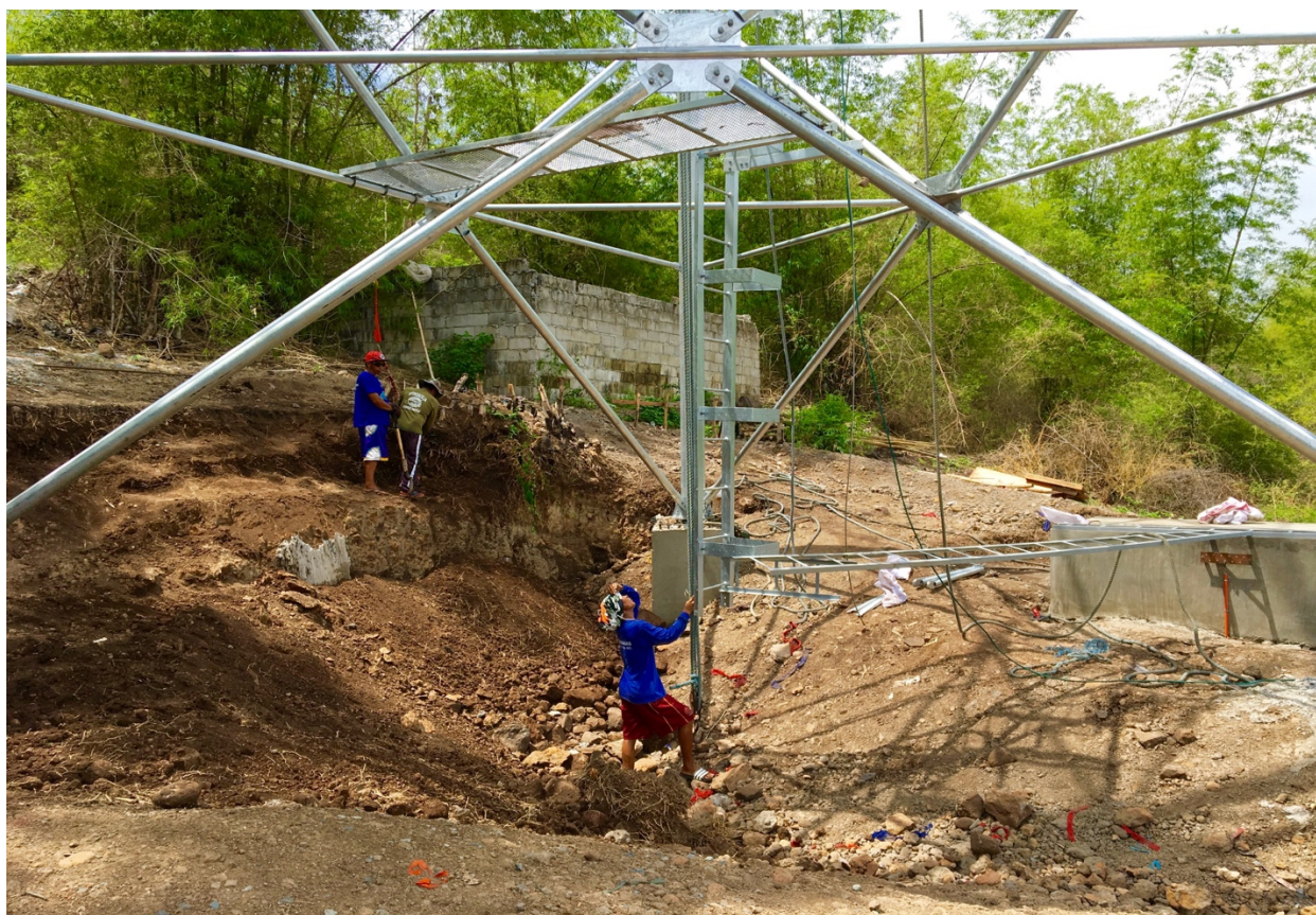
Picture 1.3. Construction such as this tower of a major telecommunication company paves the way for the influx of outsider's influences into the island. Photo: Angelito Nunag (25 May 2017).
