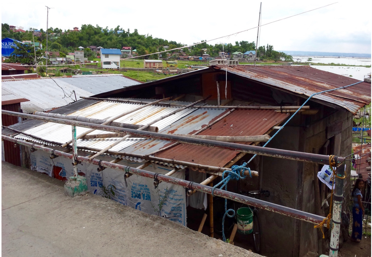
Picture 5.5. A house that is reinforced by a serga is commonplace on the island. Photo: Angelito Nunag (01 August 2015).
