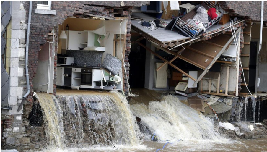
Fig. 1.5 Houses destroyed by the flood at Pepinster (Verviers) on the 16th of July (©EPA)
