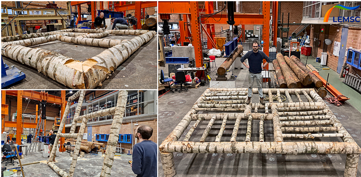
Fig. 5. Mock-up of a reciprocal log floor 4 m × 4 m, made by the authors (birch wood).
