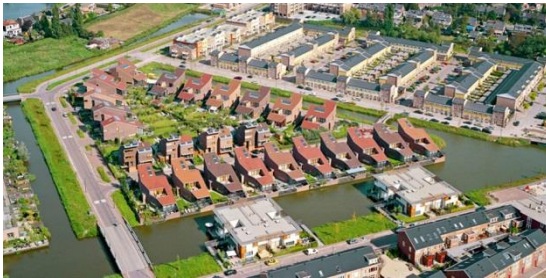
Nieuwe Terbregge – Rotterdam (1996 – 2001) 860 log. – 21,5ha
