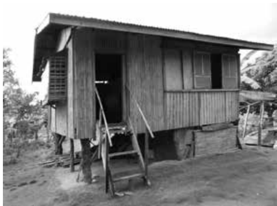
Fig. 8 House repaired and upgraded in Cuartero, 2017 © CRAterre, Dejeant F.
