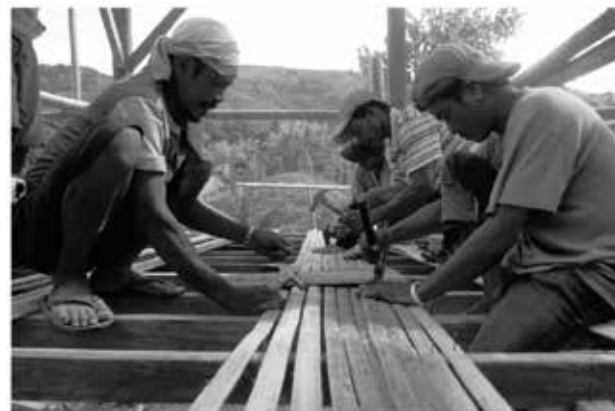
Fig. 6 On-the-job training for carpenters in Cuartero, 2016 © CRAterre, Cauderay E.
