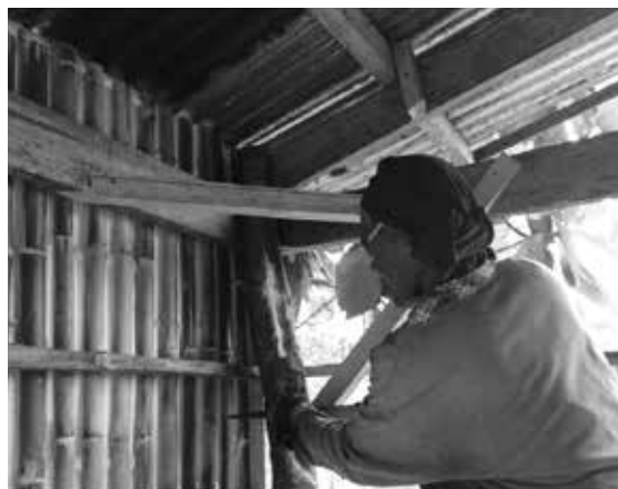
Fig. 11 Training on repair and upgrading of houses for carpenters in Cuartero, 2016 © CRAterre, Dejeant F.
