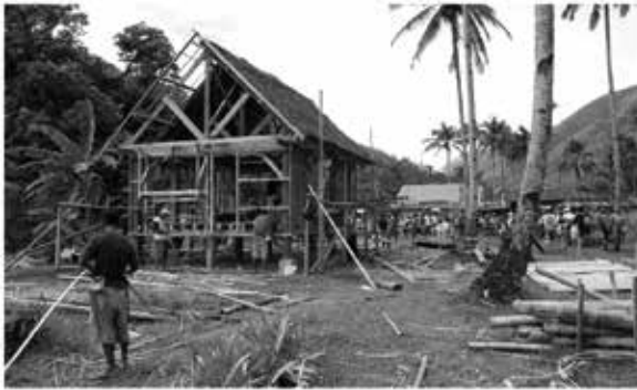
Fig. 3 Pilot house in Oyang built within the shelter project in Libacao, 2014 © CRATERre, Caimi A.
