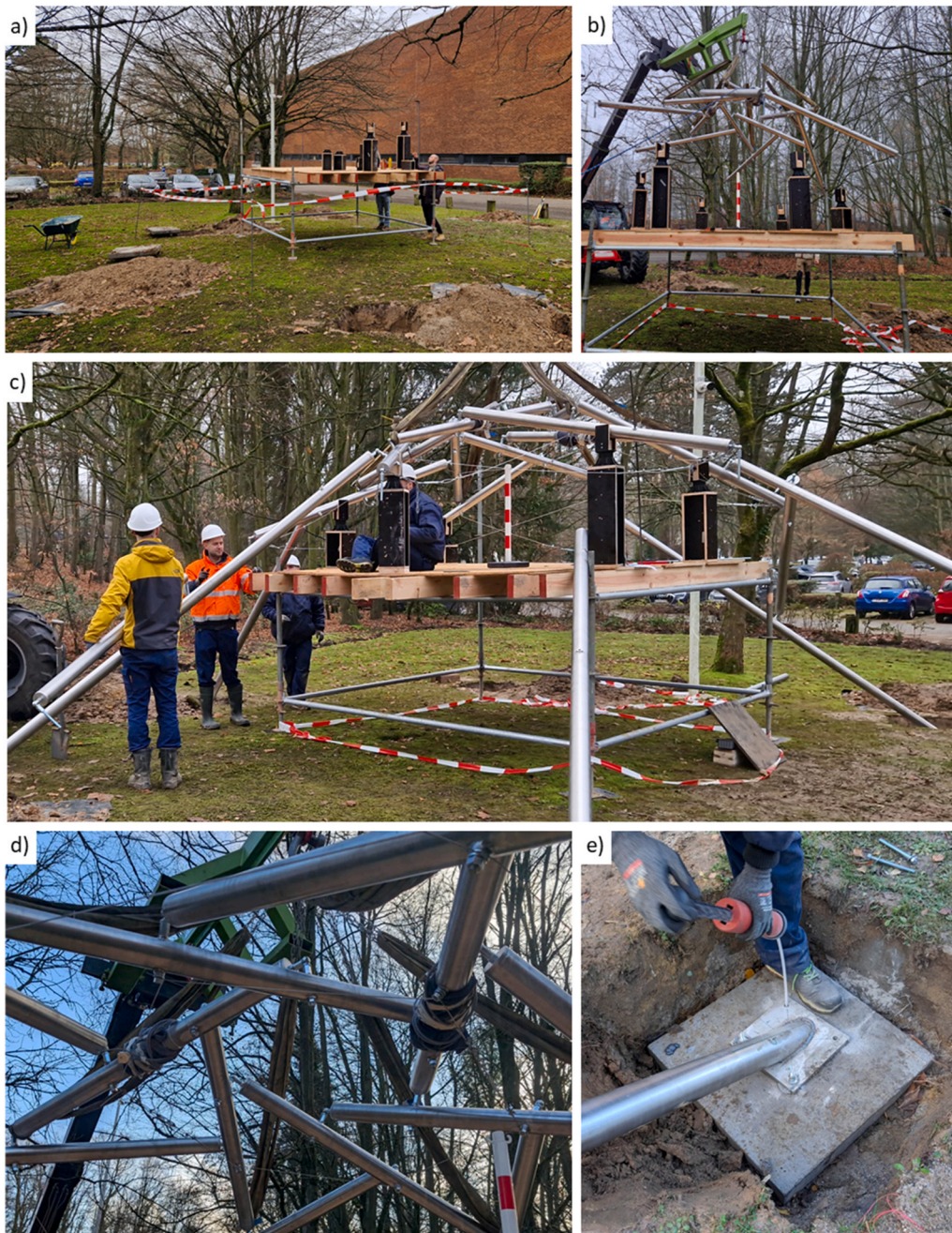
Fig. 17. a) Site preparation. b) The lifting equipment is placing the RS–12B on the temporary supports. c) Tubes of rings C and D are being installed sequentially. d) View of the central area. e) Tube supports are anchored in the concrete slabs.
