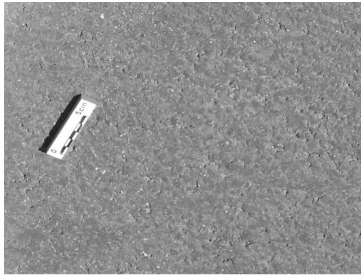
Fig. 12.12. Photograph of the road, composed of bituminous aggregates.
