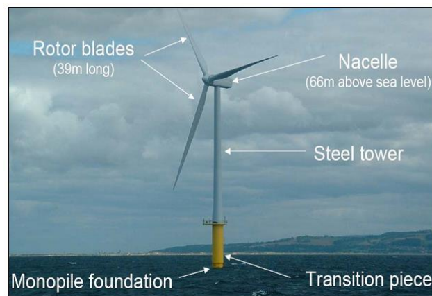
Figure 1, Wind Turbine system components
