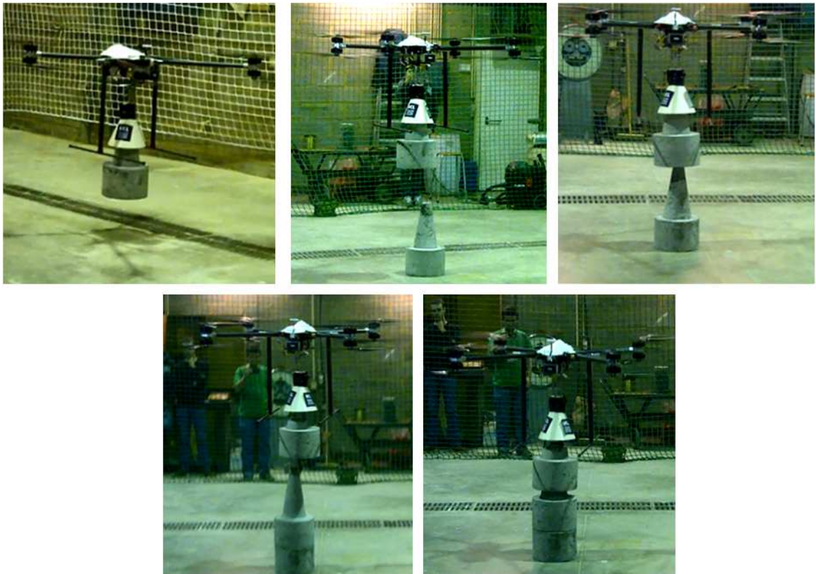
Figure 3: Construction of a column made out of concrete precast elements at the “Drone Zone” of the UCL
