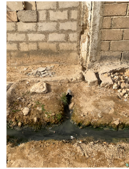
Self-dug drainage system and connection to dwelling.
