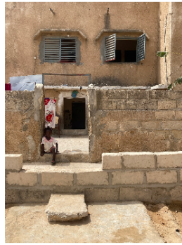
Waterproof walls in front of dwelling.
