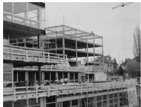
Fig. 3 - Marx Lévy, Jean-Pierre Vouga architects: Bergières school complex in Lausanne, 1969-1976, construction site (AVL, file C4-38).
