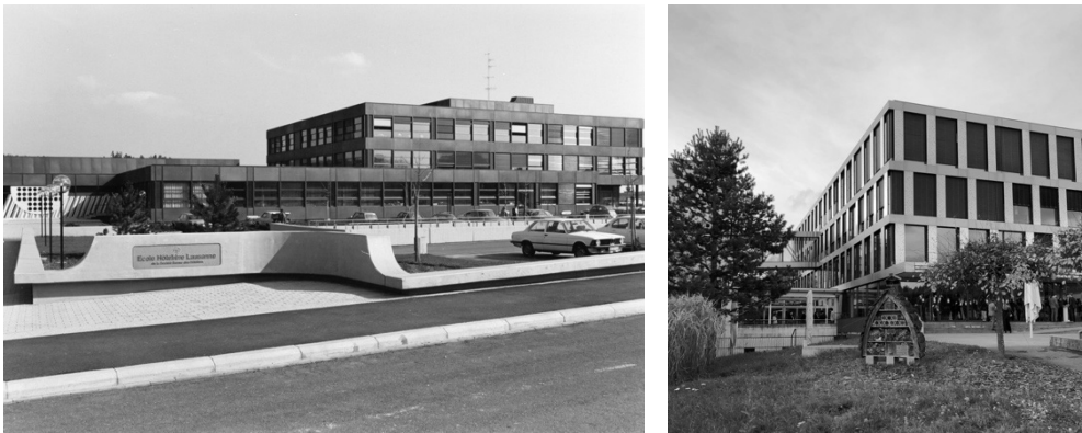
Fig. 8 - Helfer Architekten, Jacques Dumas et Serge Pittet: the École hôtelière de Lausanne, part of the CROCS programme, 1973-1976, upon completion (École hôtelière de Lausanne, historical file), and today, following an energy-efficient renovation of the building envelope that was highly destructive (picture by G. Marino) on the right.
