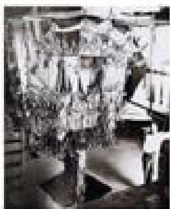
1. Antoni Gaudi's model on the suspension model for the Sagrada Familia.
