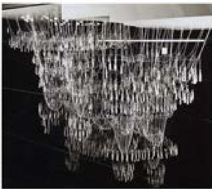
1. Antoni Gaudi's model on the suspension model for the Sagrada Familia.
