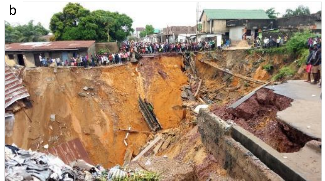
Fig.1. Destruction of infrastructure (road, houses) due to urban gully expansion. (a) Laloux gully and (b) Livulu gully in Kinshasa (December 2019).
