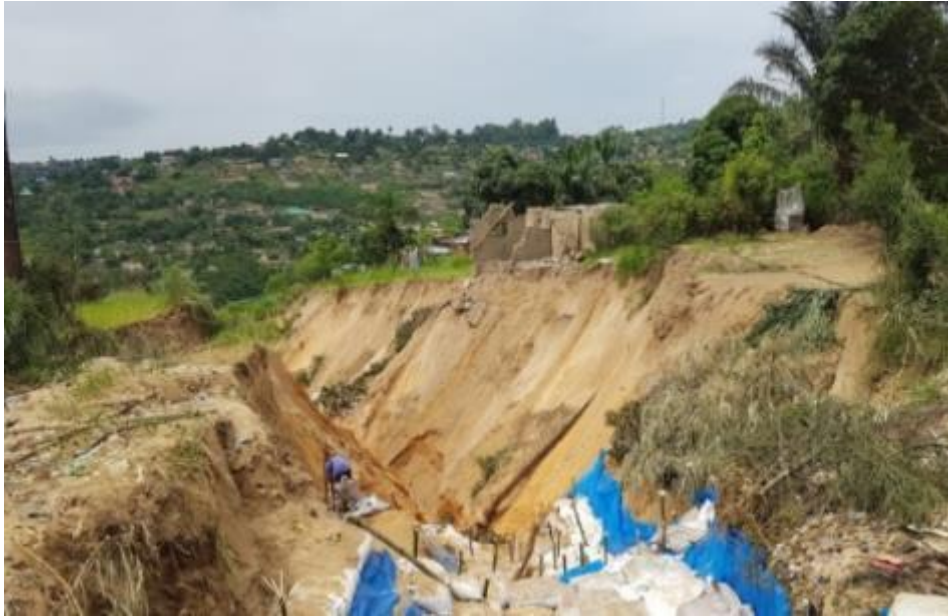
Fig. 5 Tchad gully in Kinshasa (November 2019)
