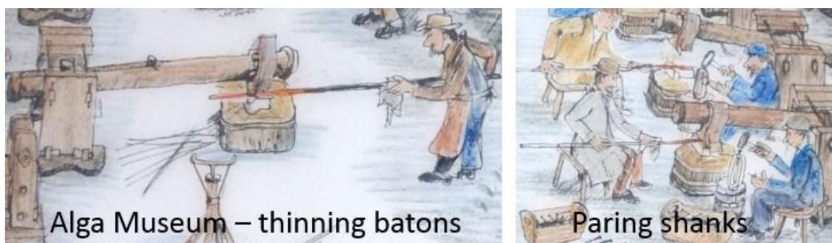
Fig. 26. The Alga nail and spike factory circa 1851. The vertical obore is shown on right, in right foreground
