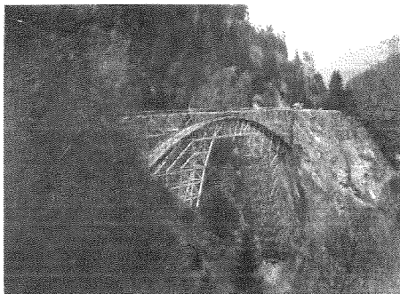
Figure 1: Salginatobel Bridge under construction [Hs 1085 1929-30-1 Salginatobel-Bruecke, ETH-Bibliothek, Archives and Private Collections, Maillart collection]
