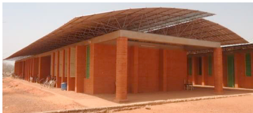
Fig.3 Construction of CEBs building
