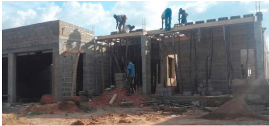
Fig.1 Construction of cement blocks dwelling in Ouagadougou
