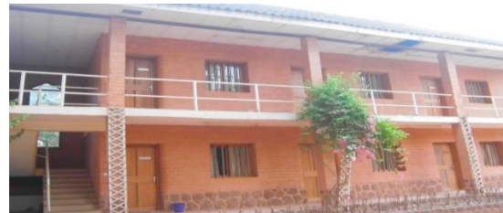
Fig.3 Construction of CEBs building
