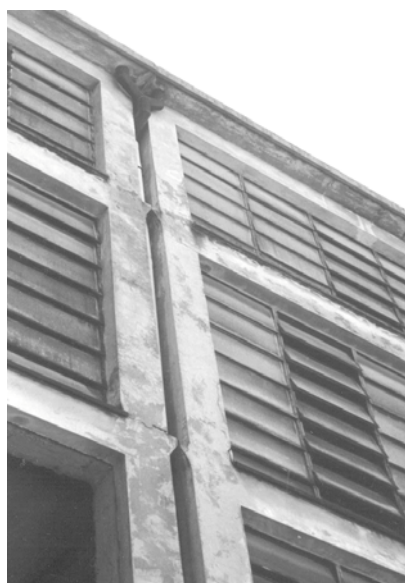
Facade: particular of the structural joint
