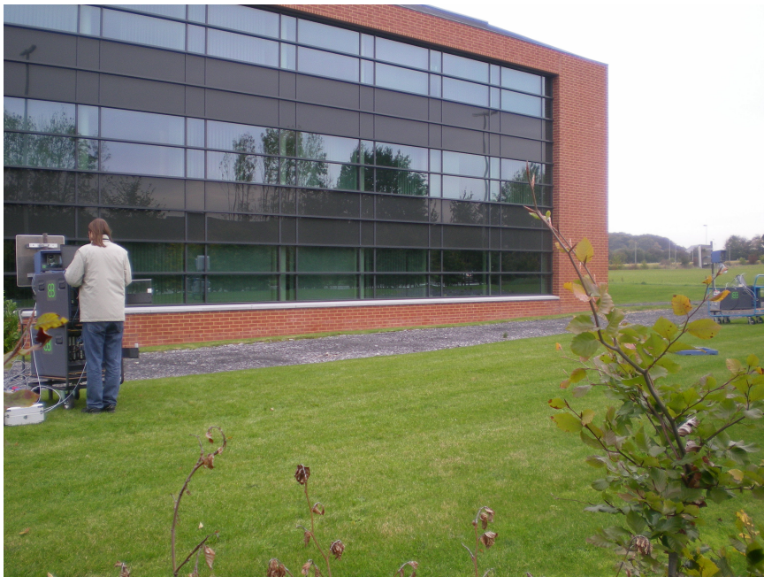
Figure 6.2: Isolated office building
