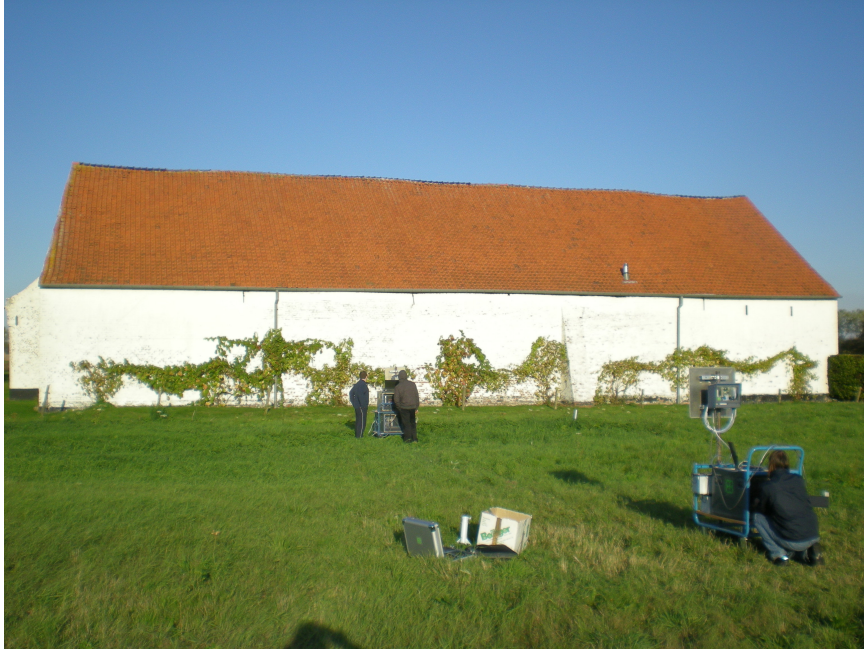
Figure 6.1: Isolated rural building
