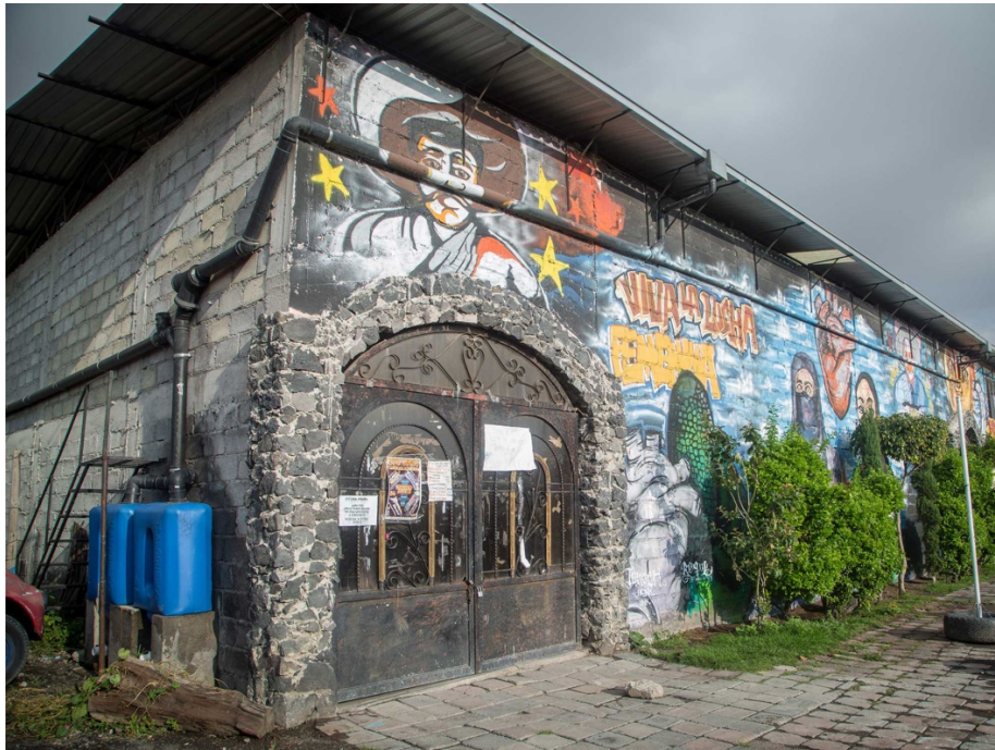
Figure 1 – Community rainwater treatment plant co-built in 2015 on a public building by the NGO Isla Urbana and the local residents in the community of Yuguelito, municipality of Iztapalapa, Mexico City. The plant can capture and purify up to 180,000 litres of water per year (© 2015 Isla Urbana with permission).
