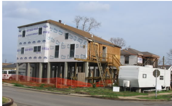
Fig. 1.8: House raised on piles in New Orleans, as a measure to mitigate flood risk.
