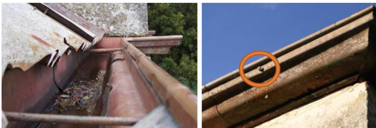
Fig. 150. Hawthorn Vale farmhouse, Koroit, showing moulded gutter and laundry nails in-situ. Author.
