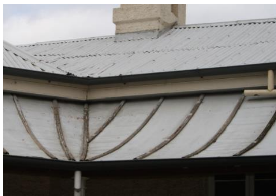
Fig.71. Flat zinc sheet roofing 1839, Woolmers Cottage, Tasmania.
