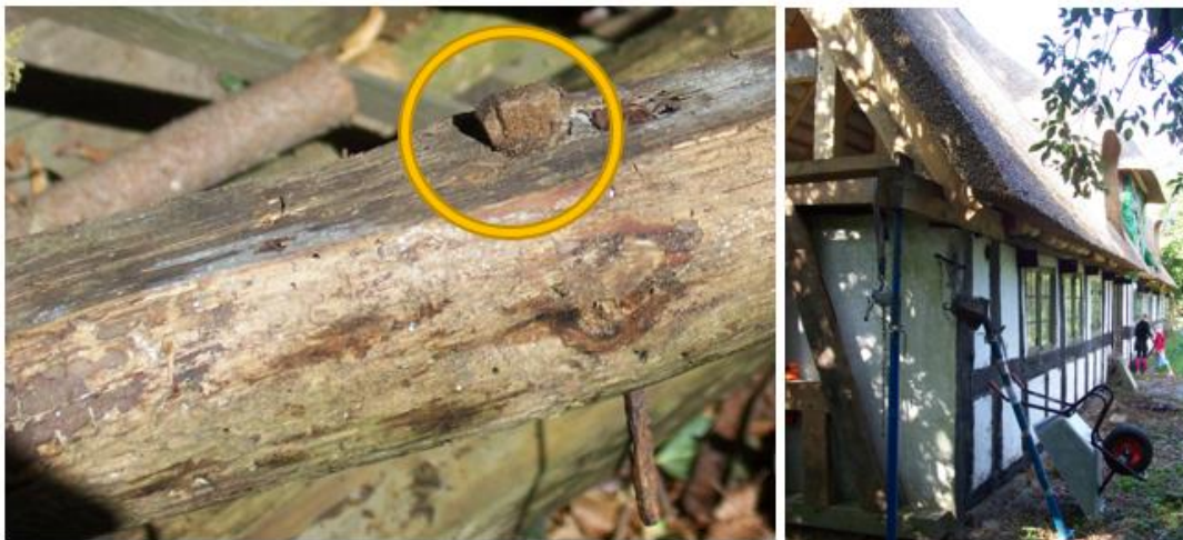
Fig. 22. Fully developed head to an oak nail, ringed in yellow, driven through fir thatching poles, squared on two sides only, and into fir rafters. A rear view of the 1560 oak frame Asferg longhouse during renovation in 2008. Author
