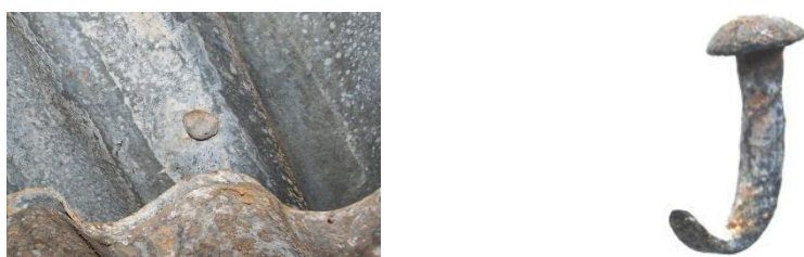
Fig.76. Side lap rivet, 'Muntham' barn, circa 1854, and clenched dog nail of type used. Author.
