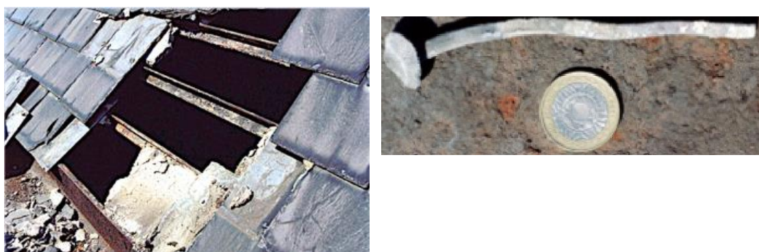
Fig. 79. Papplewick Pump Station roof repairs. The heads of the ‘lead nails’ can be seen top left, and a straightened example is shown on right. (Photos Terry Hughes).
