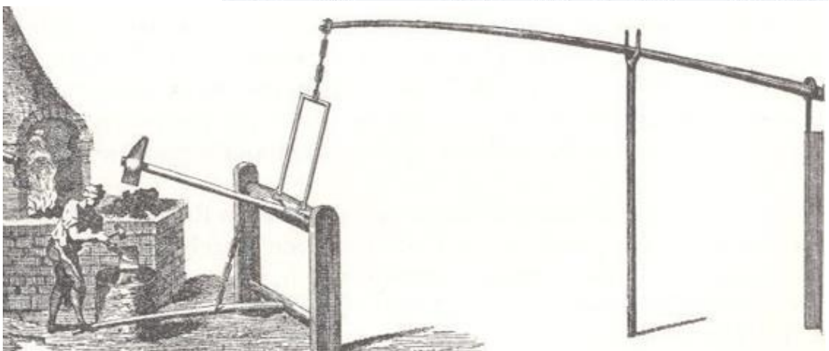
Fig. 6. First recorded in 1352, there is no image of an Oliver prior to this one of 1770, which shows its use in the cutlery industry. Flattened nail finds suggest it was in use by 1700 in forming flat lining nails. YOUNG 1770, 25
