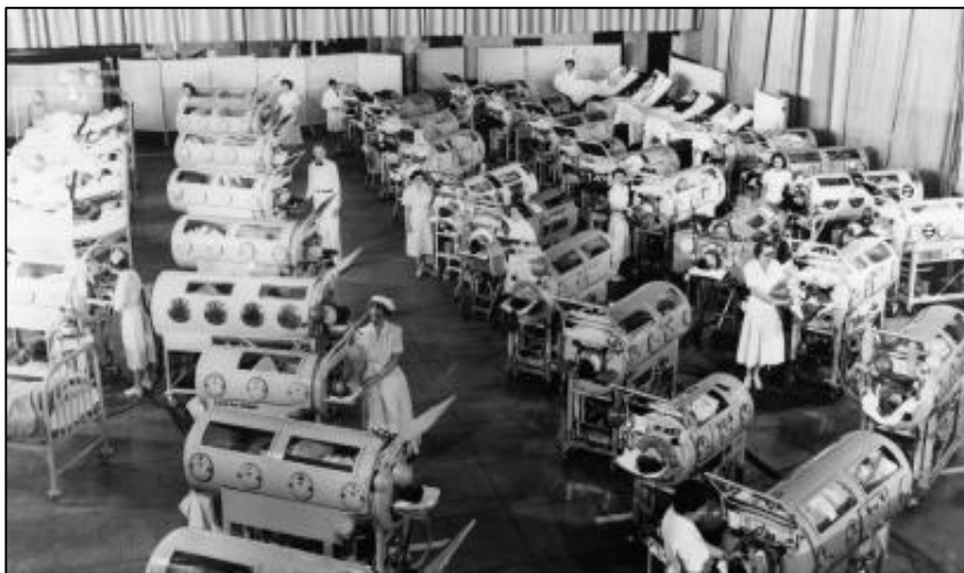
Fig. 33: Iron lung based on negative-pressure ventilation used in the treatment of polio victims during Denmark's polio epidemic in 1952, before MV era [244].
