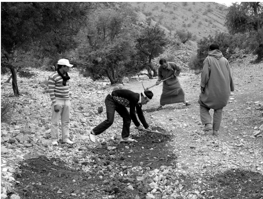
Repairing a dirt road after the rains in an isolated village
