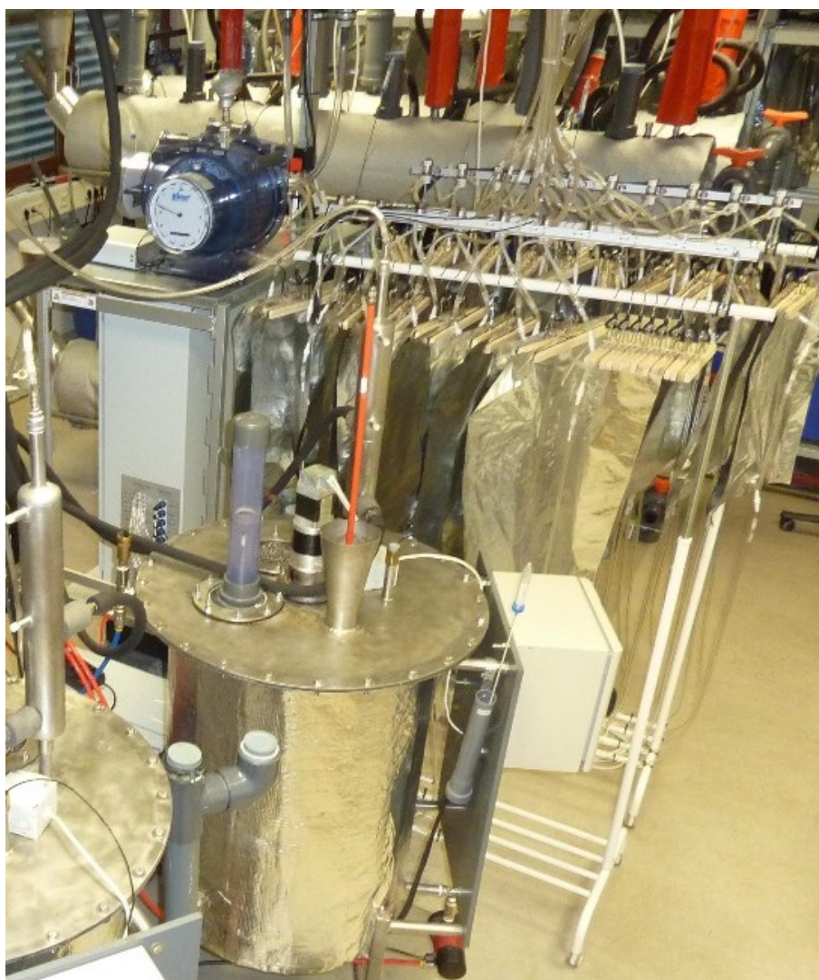
Figure A 9. Biogas monitoring system N° 2: gas bags used to store temporarily the biogas produced by the reactors.
