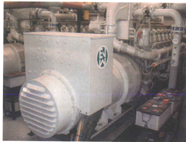
Figure 6: The CHP engine
