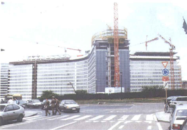
Figure 3 : The Berlaymont Structure during the building site
