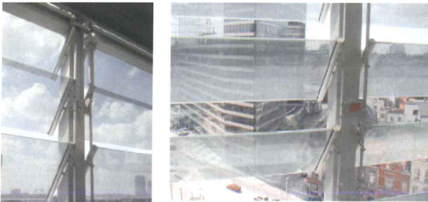
Figure 5: The movable louvers of the Façade
