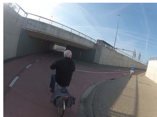
Fig. 2. A recently-built bicycle tunnel that provided a safe way to cross a busy street.
