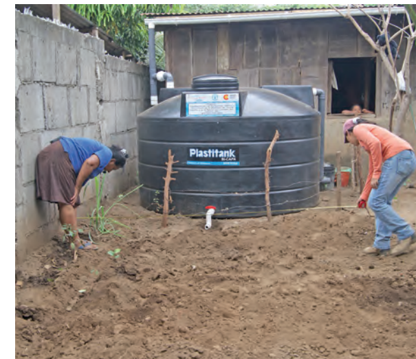
The project provided 430 rainwater harvesting systems, each linked to a 5 000 litre storage tank
