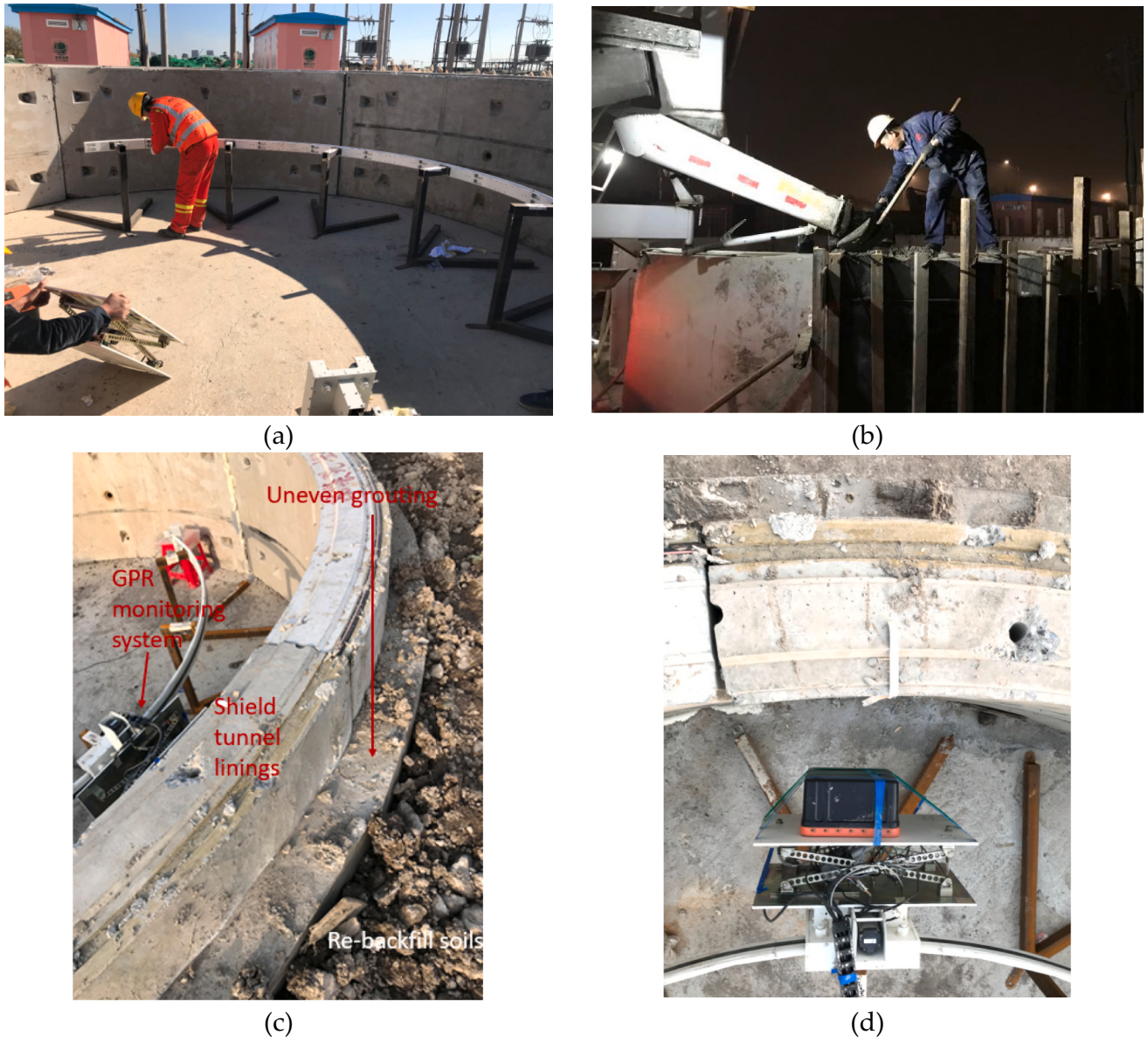
Fig. 9. The construction of the full-scaled experimental model. (a)The installation of GPR monitoring system. (b) Grouting construction. (e) The removal of wooden framework and the earthwork re-backfills. (f) The top view of GPR, tunnel linings, backfill grouting and soils.
