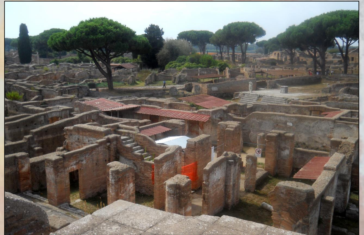
During the restoration works (2021)
