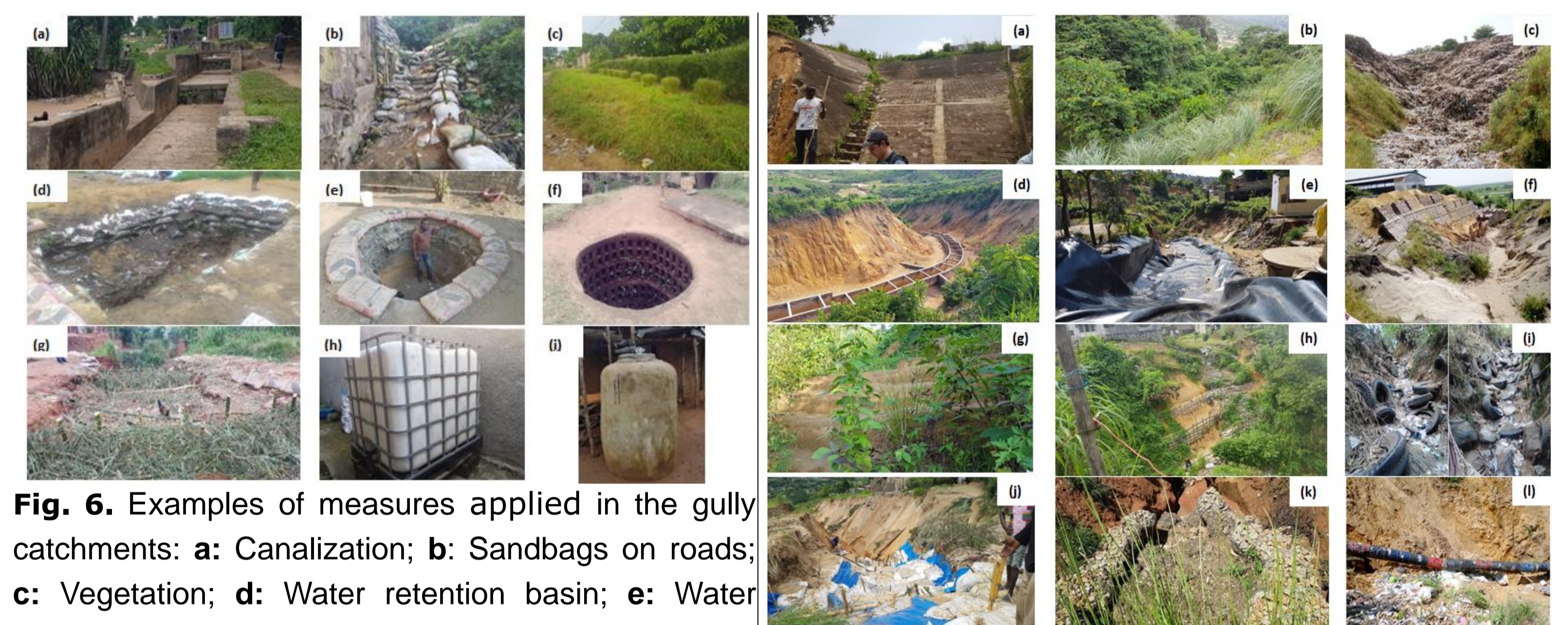
Fig. 7. Examples of measures applied in the gully head or in the channel: a: Concrete slide; b: Vegetation; c: Household waste; d & e: Channelization (with concrete and metal); f: Retaining walls; g & h: terraces (without and with protection); i: Tire dikes; j: Sandbag piling; k: Old house carpets; l: Gabion dikes (Photo credit: E. Lutete).
