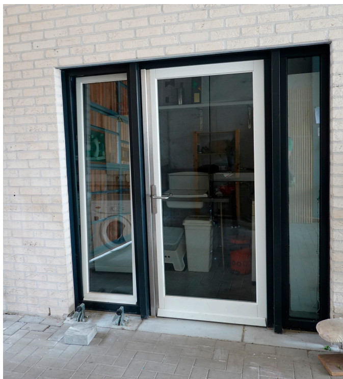
Figure 11. The communal laundry room in l'Echappée (photo by the authors, 2019).
