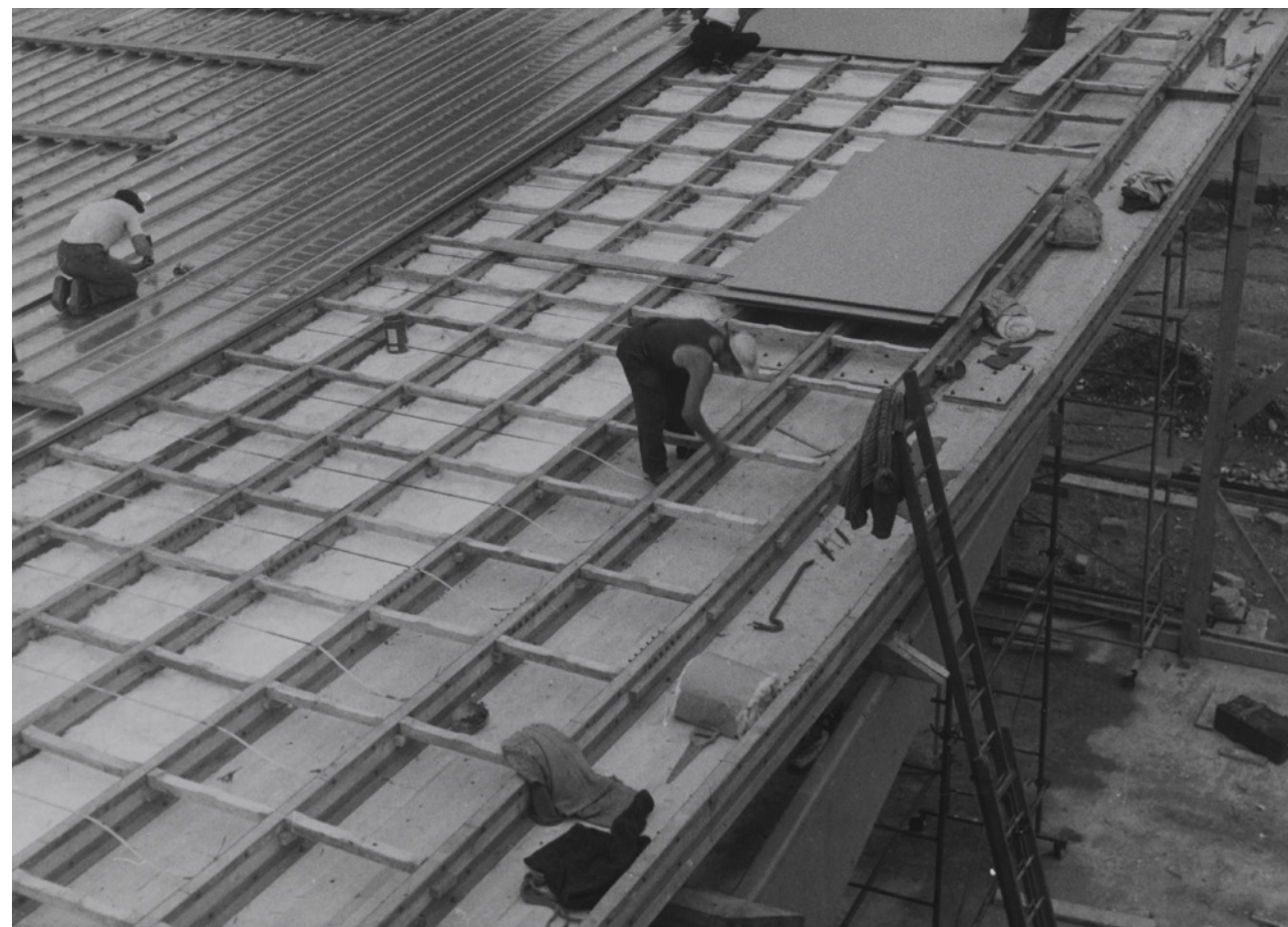
Figure 2. The Évian buvette building site in 1956: the roofing complex © MNAM-CCI, Centre G. Pompidou.
