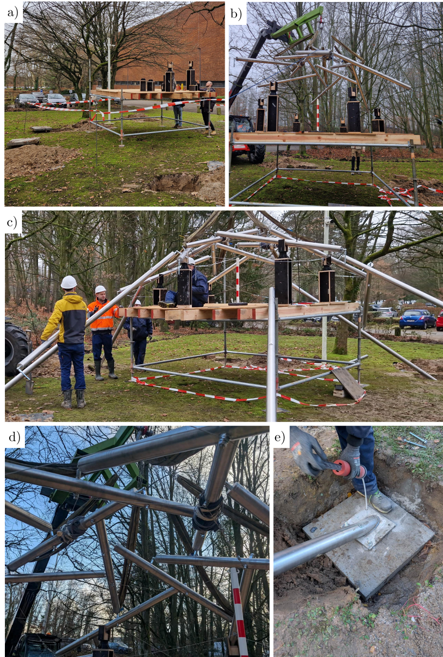
Figure 4.17: a) Site preparation. b) The lifting equipment is placing the RS-12B on the temporary supports. c) Tubes of rings C and D are being installed sequentially. d) View of the central area. e) Tube supports are anchored in the concrete slabs.
