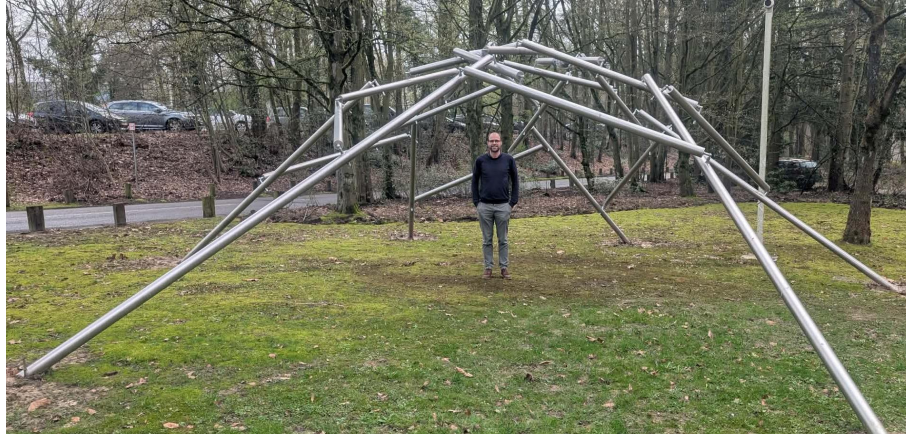
Figure 4.1: General view of the RS-24B prototype, built outdoors.
