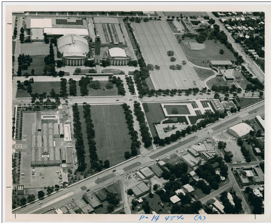
Figure 10: Aerial view of the site during construction of the Kimbell Museum of Art (lower left), taken sometime around 1968 [Source: University of North Texas Library].
