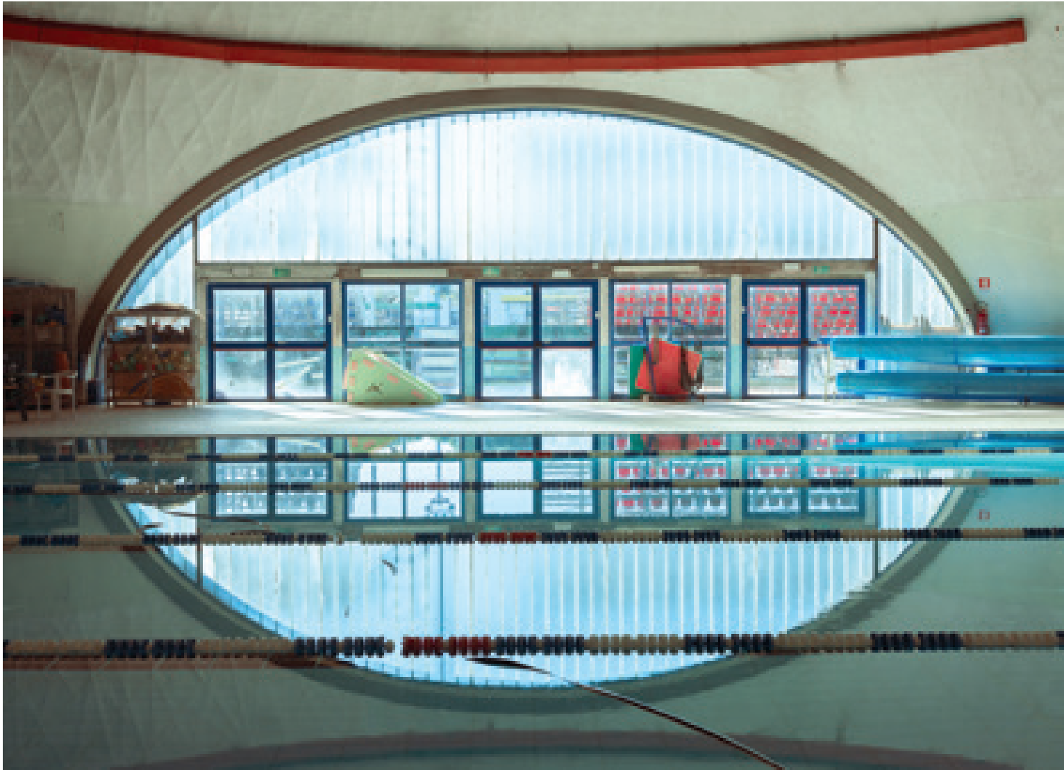
Marco Meozzi, Municipal Swimming Pool, Iolo, Italy, 1976 (Binishell System Application Example)
