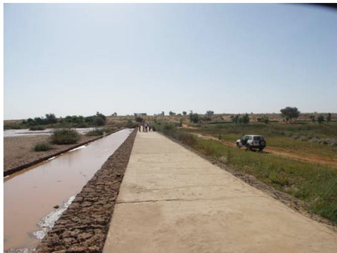
Figure 3-10: A small dam impedes runoff from the Mare de Kouana that is located upstream in the kori, on the left hand side of the dam. While upstream stagnant water is present, downstream, on the right hand side of the dam, the kori is already dry and densely vegetated (photo: E. Bartholomé).
