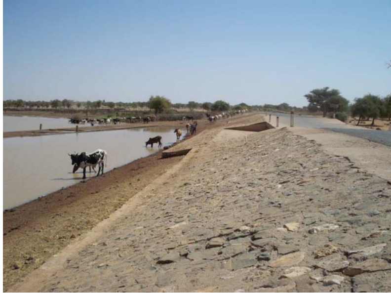
Figure 3-18: A road dam on the road to Tera in the town of Dargol (13° 55' 20" N, 1° 14' 57" E) that retains water arriving in a small tributary of the Dargol River.
