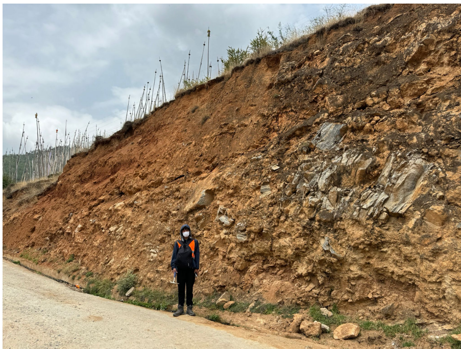
Landslide deposits in Buthan.
