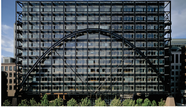
Figure 3.8 – SOM’s Exchange House in London [SOM]
