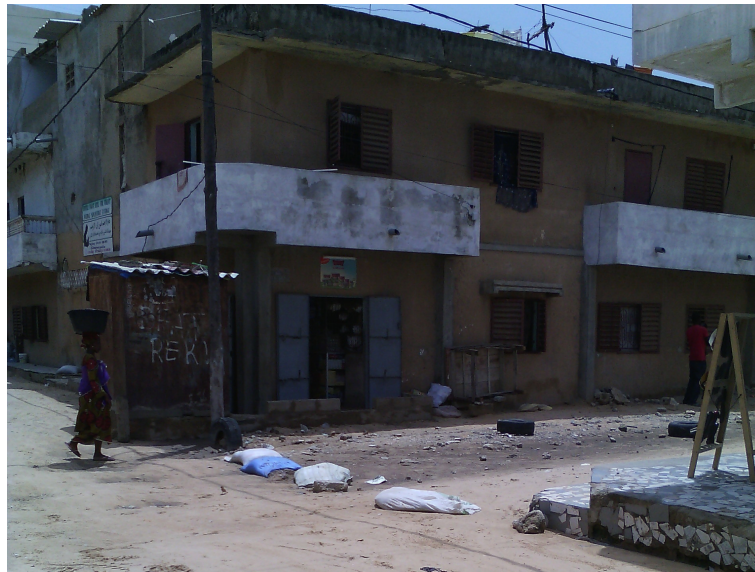
Figure 10.10: Sand Sacks in Fith Mith
