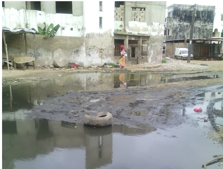
Figure 10.7: Stagnant Water in Dalifort
