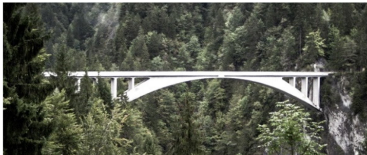
Fig. 1 Salginatobel Bridge (1929) from Robert Maillart, picture taken by D. Zastavni (2022)
