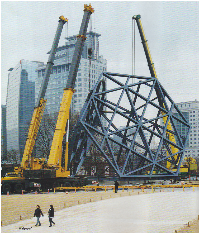
PRADA_ Transformer. Rem Koohaas (2009)
