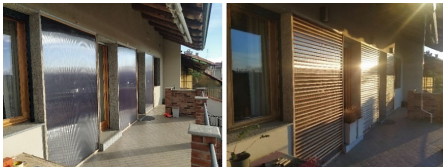
Fig. 1 Picture of polycarbonate Trombe walls developed by the authors and integrated in a real building under monitoring. (Left) Trombe walls without lamella; (right) Trombe wall with wooden lamella
