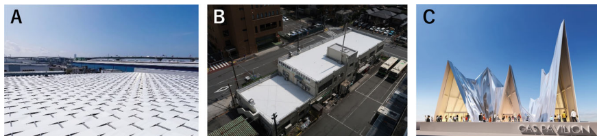
Fig. 4 Examples of radiative cooling material applications in buildings. a Roof shade method. b Waterproof sheet method (roofing method): a case where 600 m 2 was installed for the Tokyo Metropolitan Bureau of Transportation. c Concept image of the gas pavilion made with radiative cooling material
