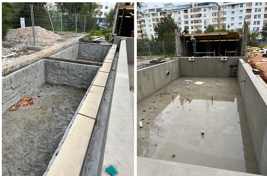
Fig. 3 Construction phase: main tank, secondary tanks and machine room
