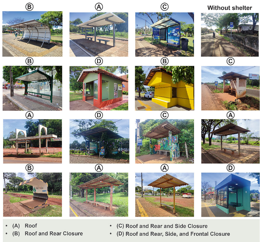
Fig. 1 Examples of bus shelters found in Foz do Iguaçu
